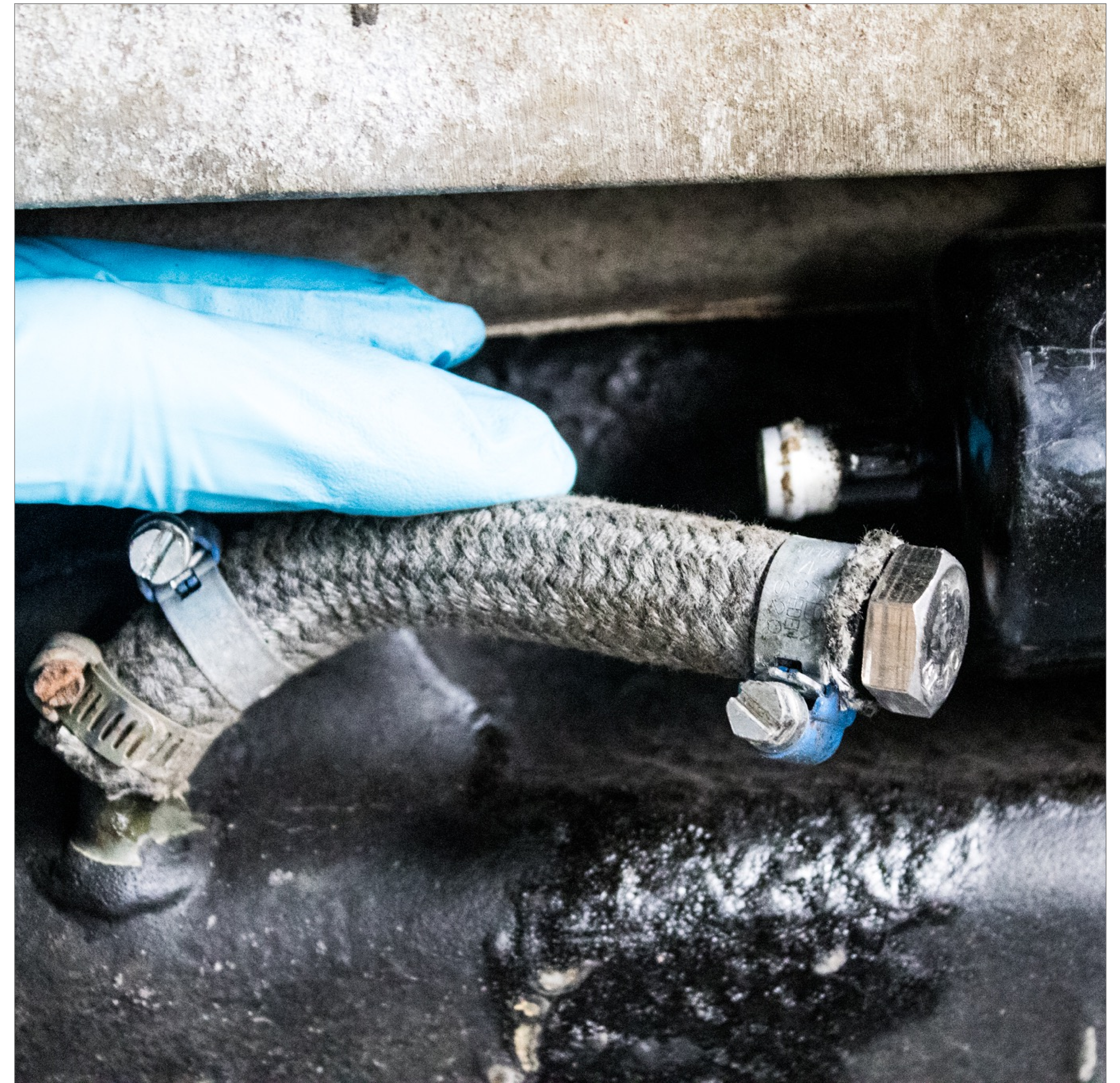
Plug off any pipes if possible, as some fuel residue may still spill from tank.
